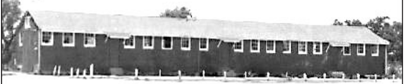
The old Scott's Branch School is shown in the top photograph. After the 1951 District Court ruling that facilities were not equal, the school was said to be 'equalized' by the addition of the classrooms shown in the lower photograph.
