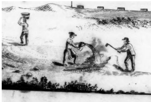
Figure 4: Historical illustration of slaking quicklime to make tabby (“Observations on the Art of Making the Composition called Tapia,” Alexander Macomb, 1811)
